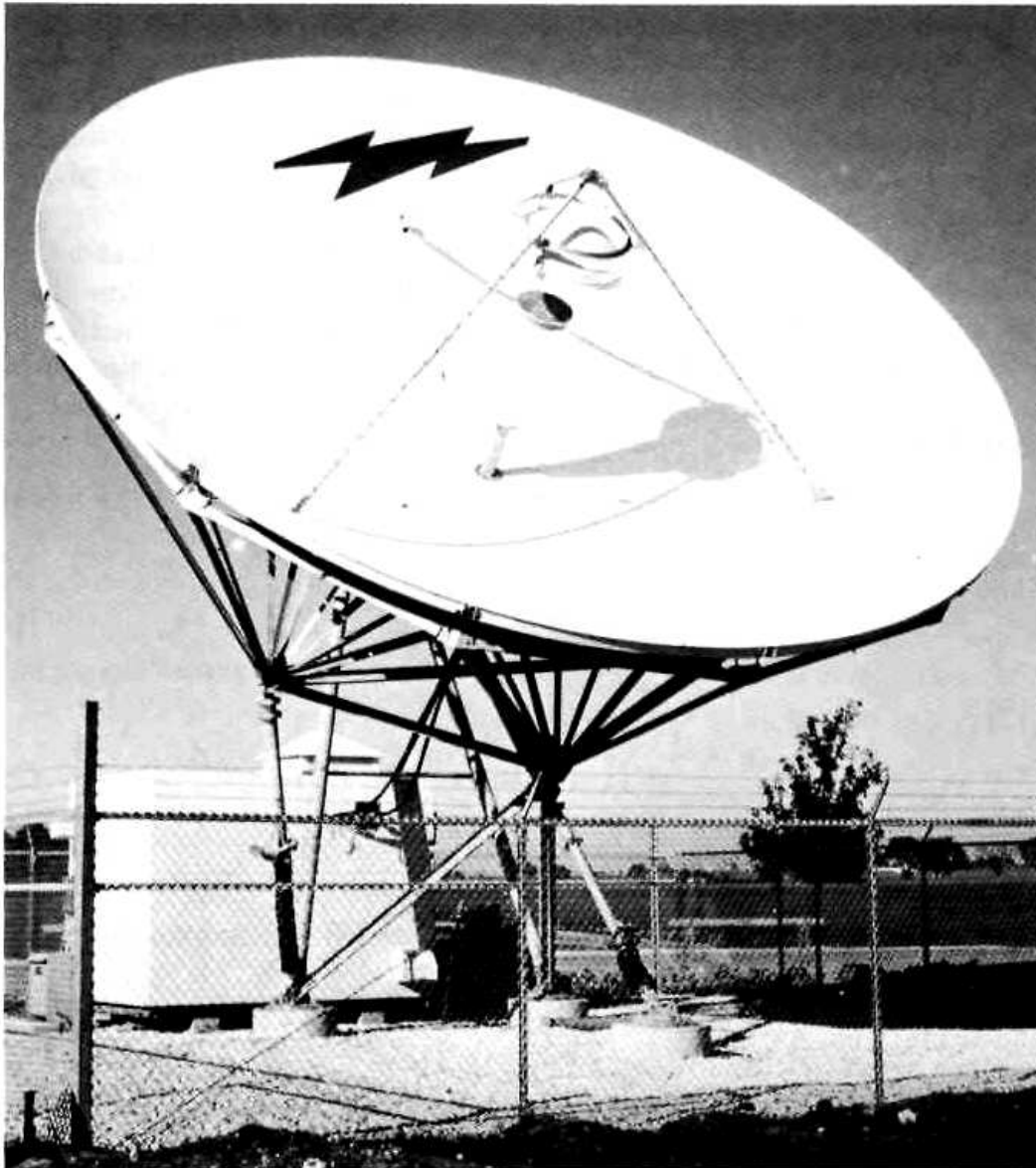
Figure 15.9 Shaped 10-m earth station dual-reflector antenna (courtesy Andrew Corp.).
