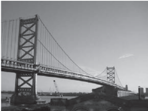
Figure 22.6.2: Ben Franklin Bridge.
